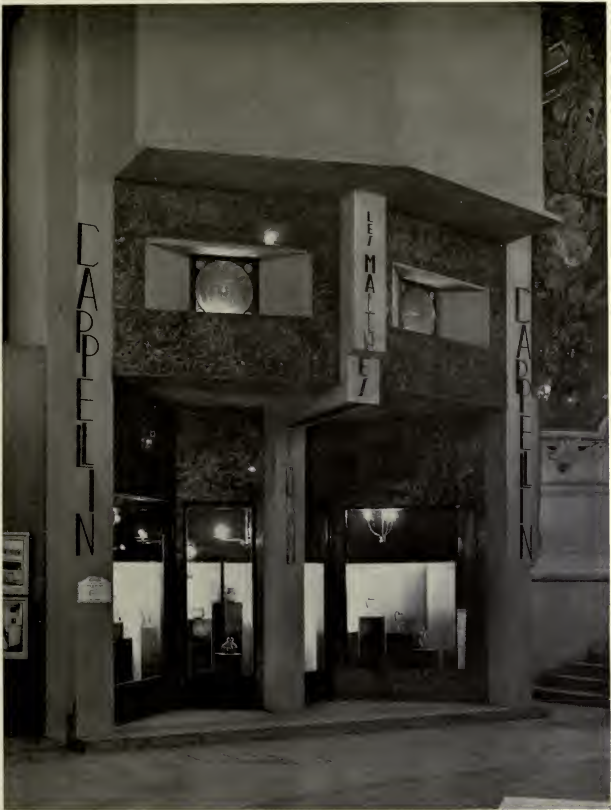
Exhibition pavilion of Cappellin's Venetian Glass, Salon d'Automne, showing the reverse effect of our modern step-back structures. While our buildings draw the eyes of the observer upward, this effect centres the attention on the most recessed inner part where the brilliant glass is attractively displayed. Designed by André Laroche-Garrus.
